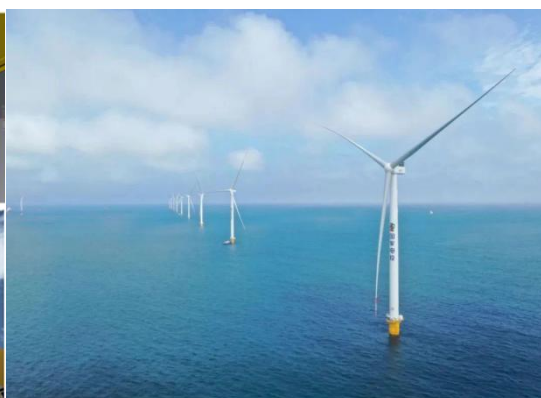
Figure 5 SPIC's offshore wind power base in Shandong Peninsula
