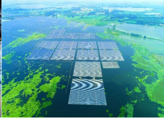
Figure 2 World's first floating PV project (Huainan, Anhui Province)
