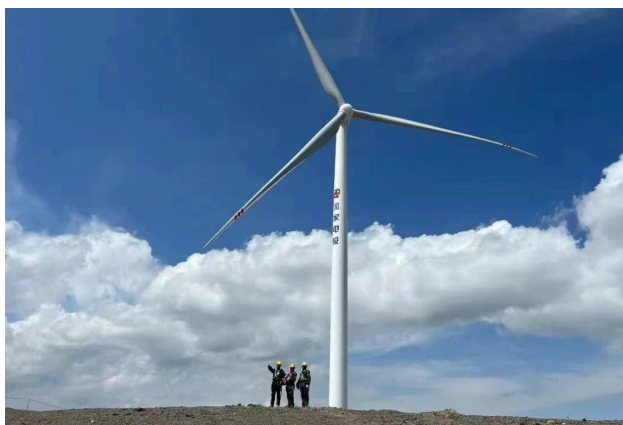
Figure 8 The first distributed wind farm in Xinjiang (SPIC's 2.8 MW wind power project in Turpan)
