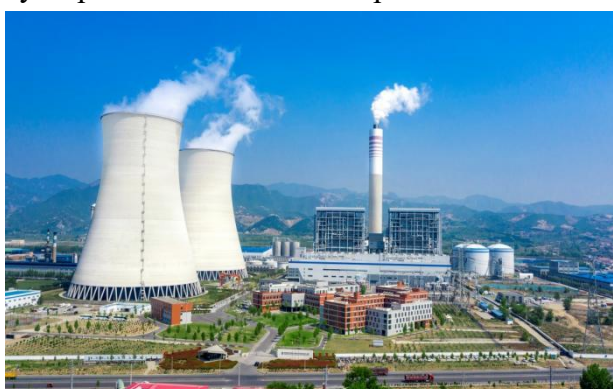
Figure 9 Two 1 GW supercritical thermal power units in SPIC's Qinyang plant, with coal consumption being 273g/kWh
