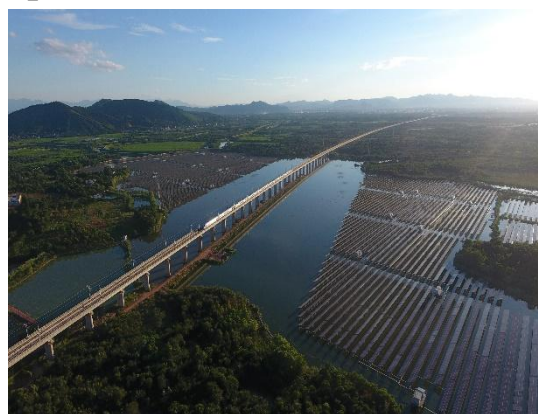
Fig. 11 Anji Caodang Photovoltaic and Fishing Pond
