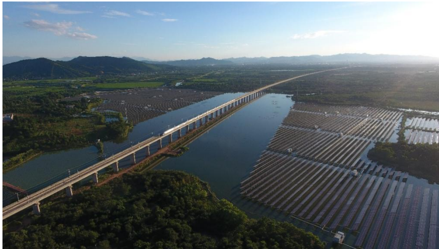
Fig. 4-6 Project Integrating Freshwater Aquaculture and Photovoltaic Power Generation in Caodang Village, Anji County
