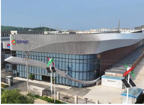
Fig. 4-2 Lead-carbon Energy Storage Station Project
