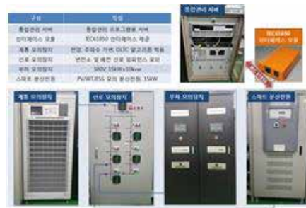
▲ Smart Distributed Power and Integrated Management System Test Environments
