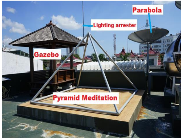
Flat roof at 4 th floor
