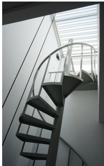
1 ST VOID AT 3 RD FLOOR
