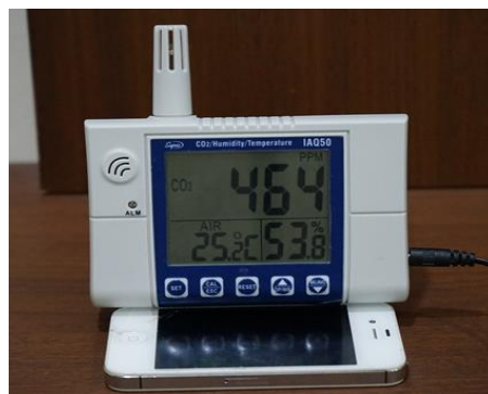
Figure 29: one person attends In air conditioned area
