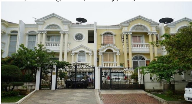
Figure 2. Typical buildings in metropolitan Jakarta.
