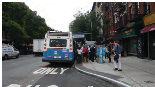
FIGURE 5 Bus bulb in Manhattan.
