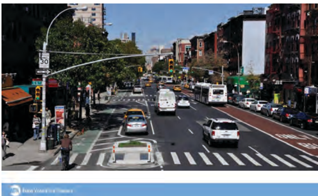
FIGURE 7 Offset bus-only lane on First Avenue in Manhattan.
