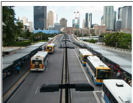
Figure 5: Cultural Centre Busway Station, South Bank, Brisbane, Australia. Photo: Breakthrough Technologies Institute.
